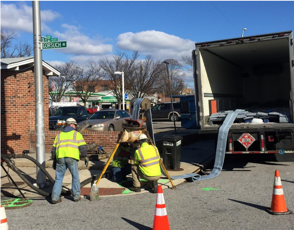
SC 976 – CIPP Liner Installation
